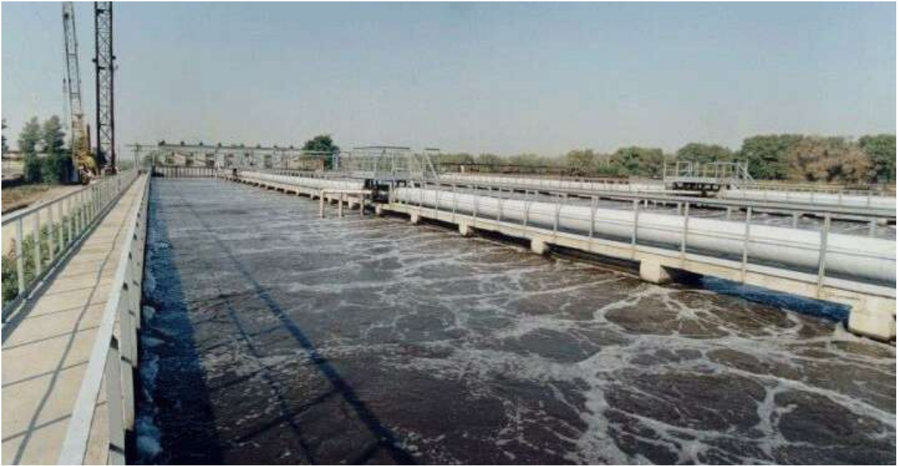
Photo 7. Aeration tanks of the first line sewage treatment facilities in the city of Rostov-on-Don after reconstruction
