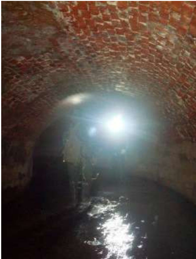
Figure 3. The main sewer (1998)
